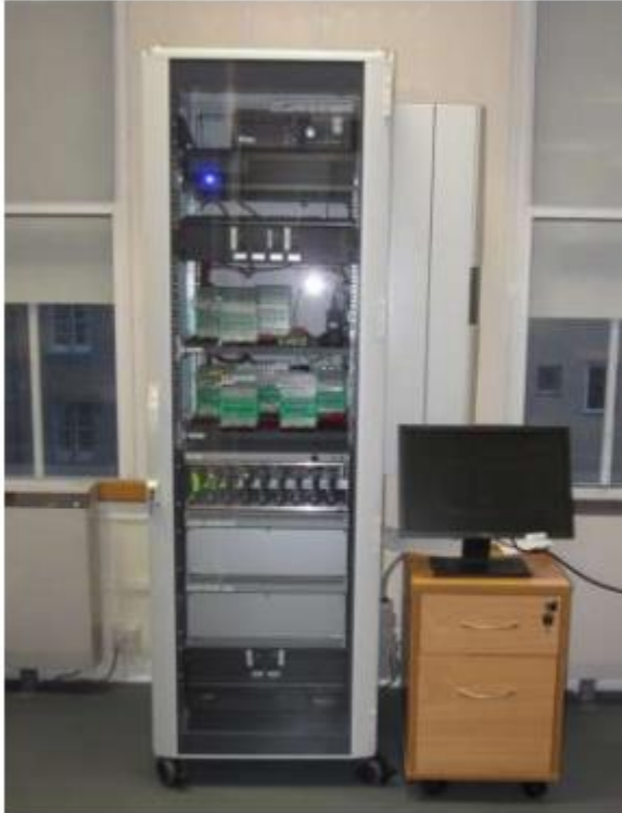
Reliability Test Station (banks of 8 sensors)
