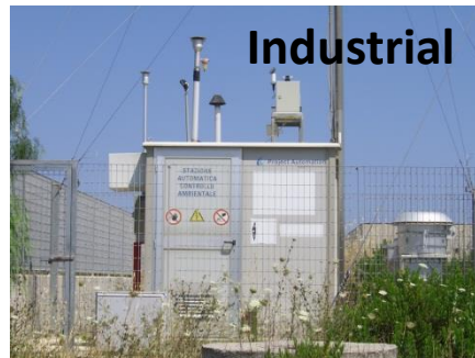
AQ monitoring station by ARPA-PUGLIA, IT
